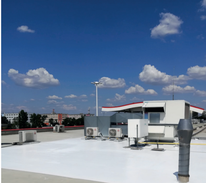
Sample surfaces treated with Egrokorr IR reflective coating:
